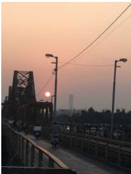
Long Bien Bridge in Hanoi on Peter's cycle path to work, built by the French during the colonial times
